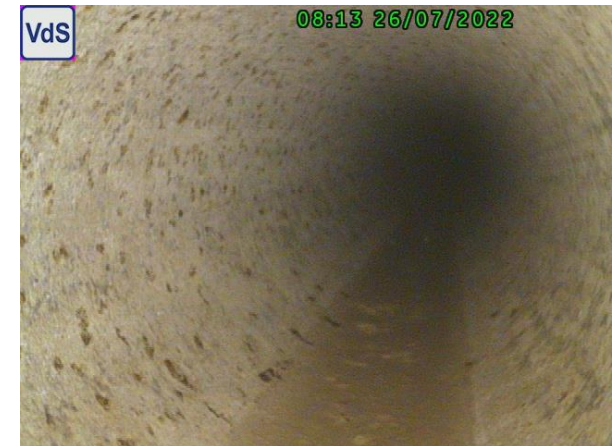
General Corrosion
