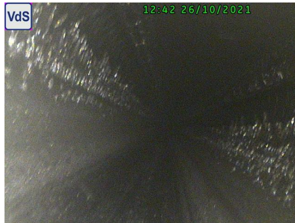
Typical air - water line
